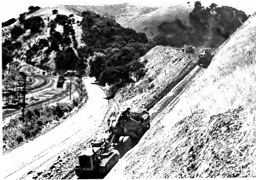
Excavating cut for new alignment. Old road shown at left
